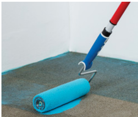
First coat application of Mapeproof Primer
