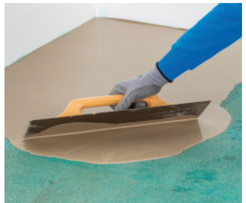
Self-levelling compound application on Mapeproof Primer
