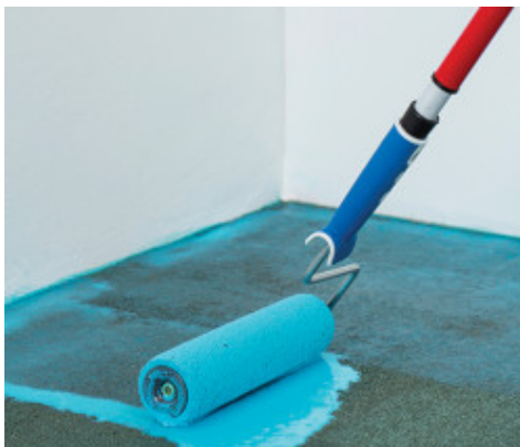
Second coat application of Mapeproof Primer
