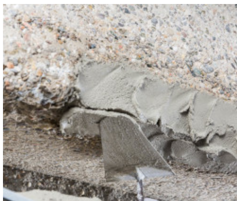
Applying Planitop Smooth & Repair R4 Zero
