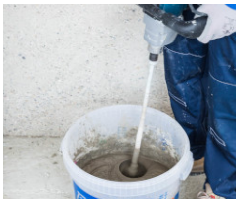
Mixing Planitop Smooth & Repair R4 Zero
