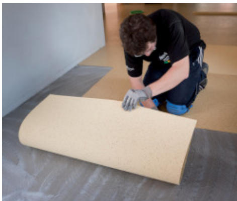
Installation of rubber tiles
