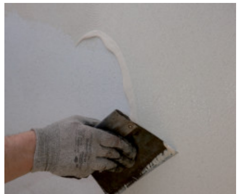
Application of Ultrabond Eco V4 SP Fiber on a wall
