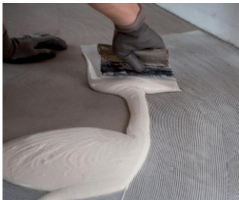
Application of Ultrabond Eco V4 SP Fiber on a substrate
