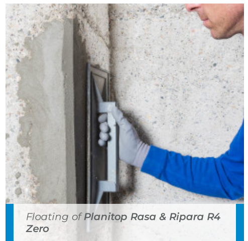
Application of Planitop Rasa & Ripara R4 Zero
