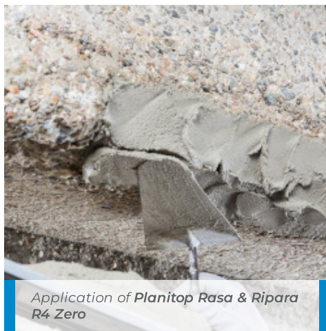
Floating of Planitop Rasa & Ripara R4 Zero
